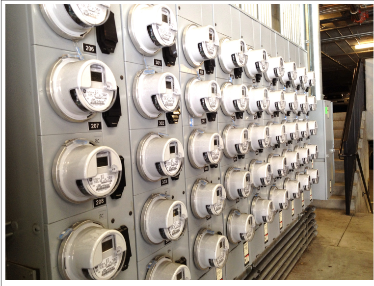
Figure 1-3. This wall of smart meters reports a granular view of energy usage for a utility company. Sensor data is becoming a huge source of valuable information that can be analyzed through machine learning techniques such as anomaly detection.
